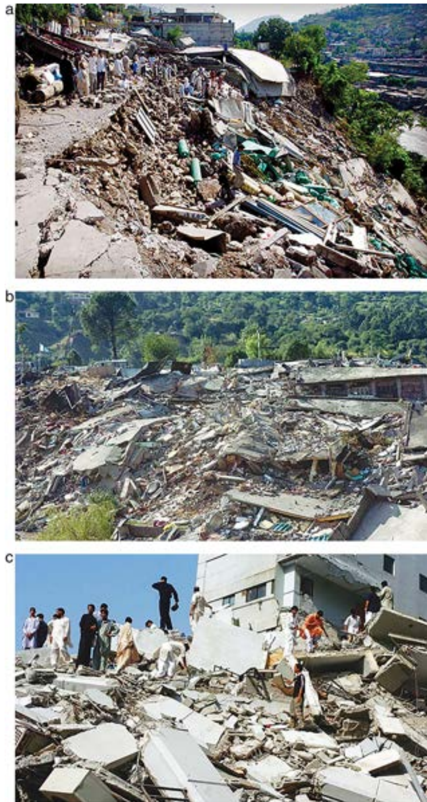
Figure 1a, 1b, 1c – Pakistan earthquake (2005) 21
